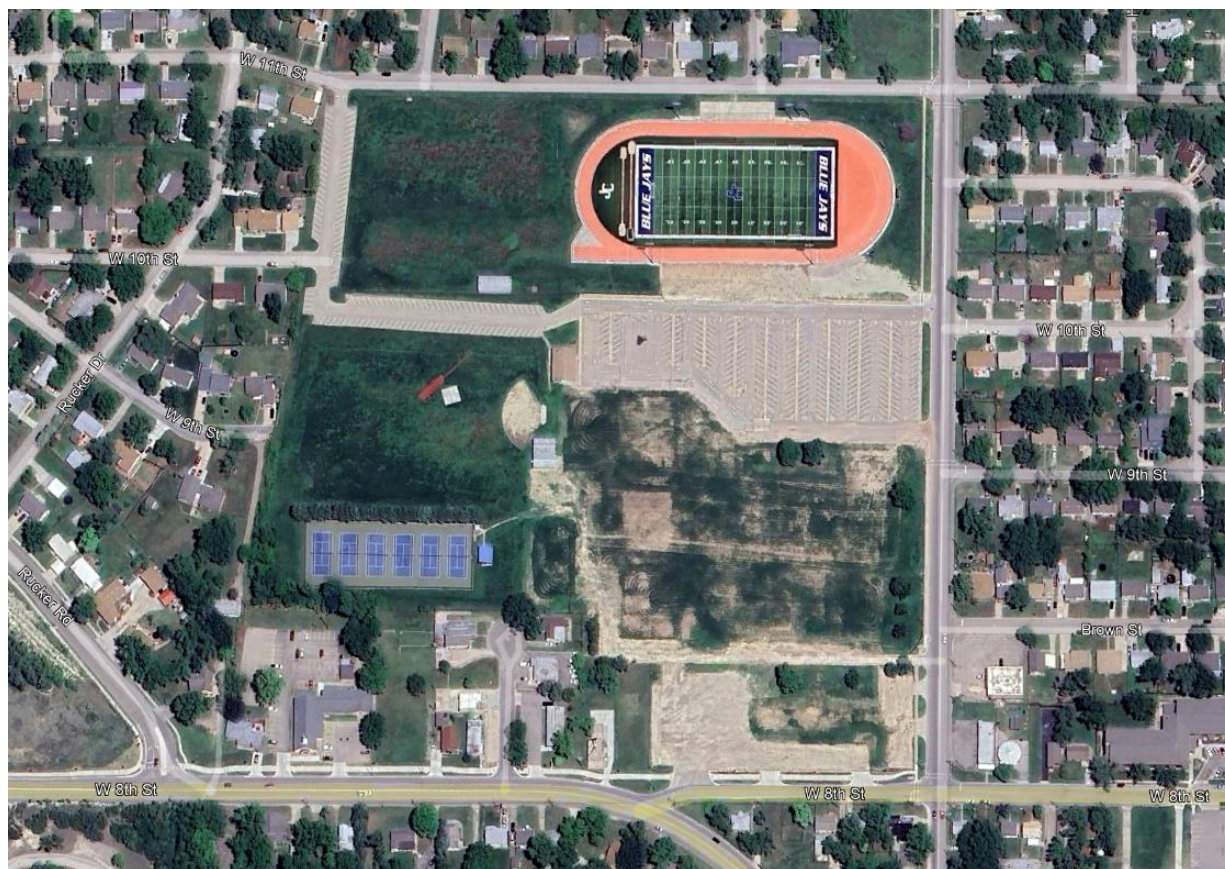
Figure 2-2: Aerial after demolition of old high school
