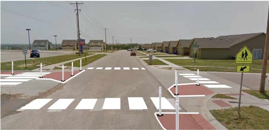
Figure 21: Hickory Lane & Clover Drive Curb Extensions
