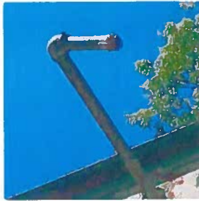
After adding a pipe screen to the overflow pipe
