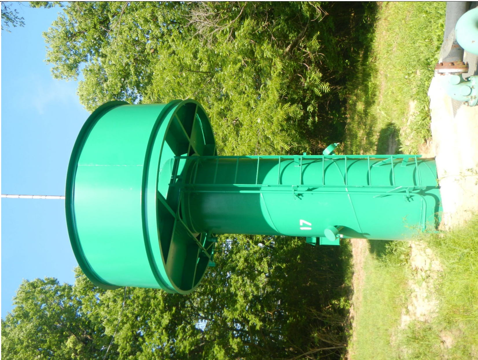
Overview of well #17
