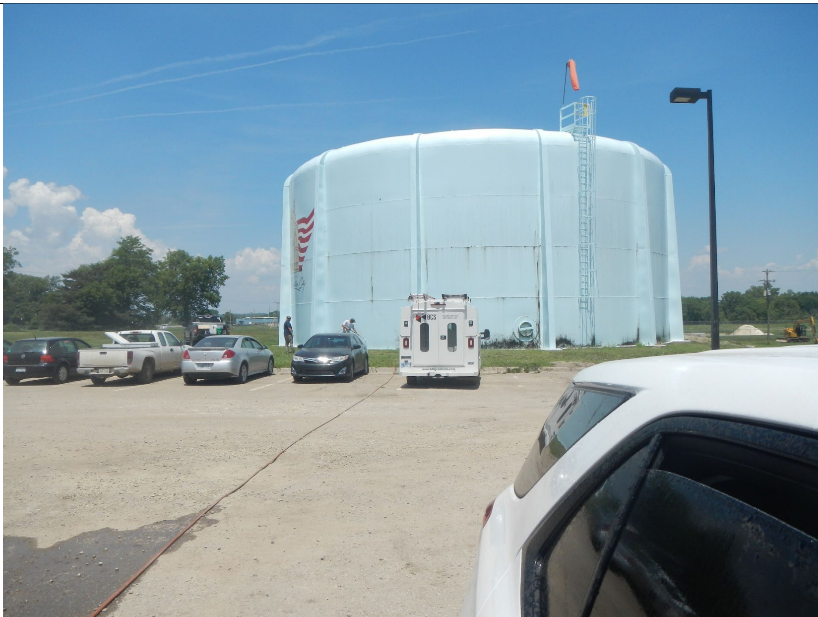
Finished water ground storage tank at water plant. Facility personnel had started to power wash mildew off tank prior to the end of the inspection.
