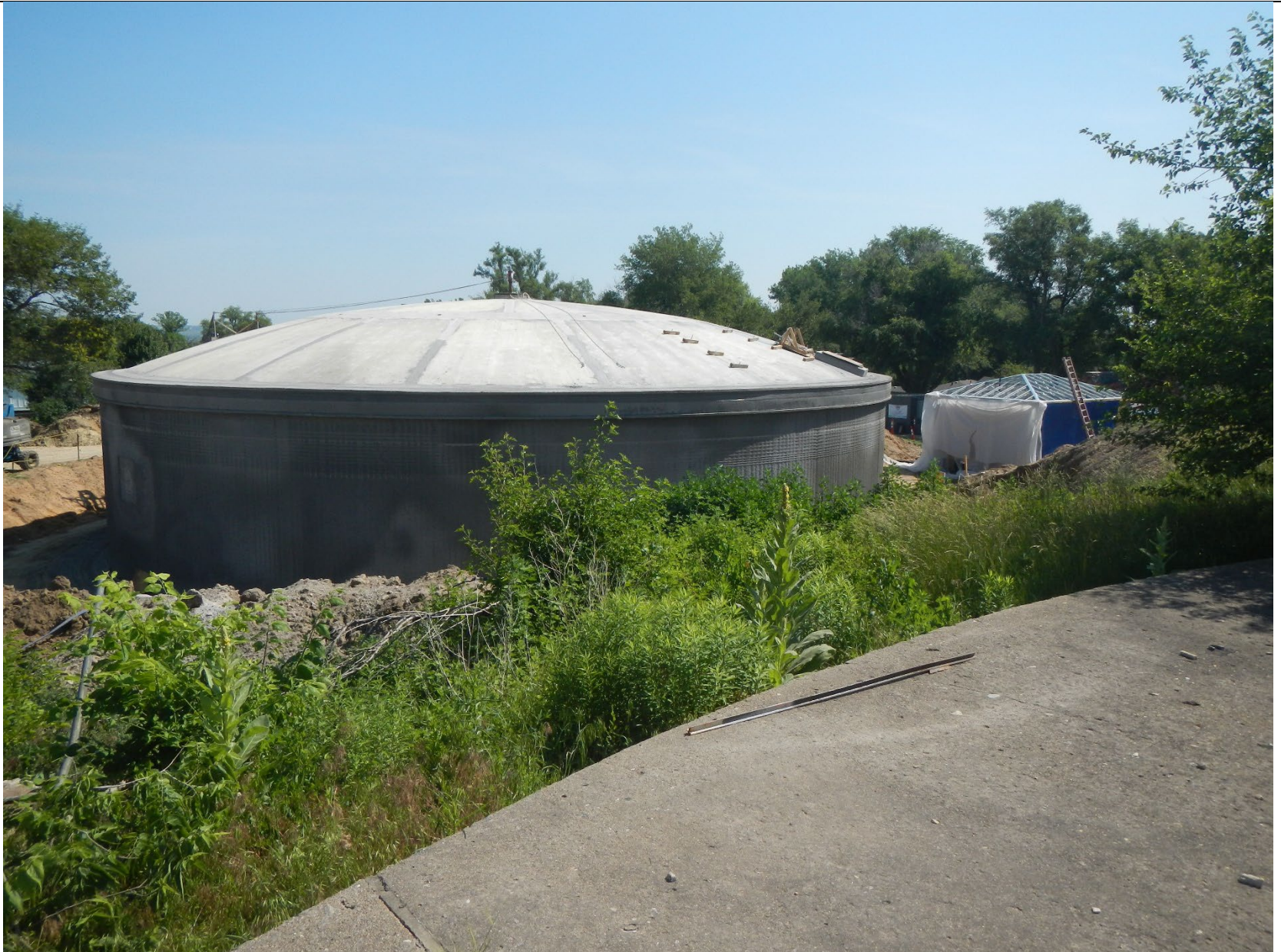
Overview of new north ground storage tank that was being constructed at the time of inspection. Building being built to the right of the tank is the new booster station.
