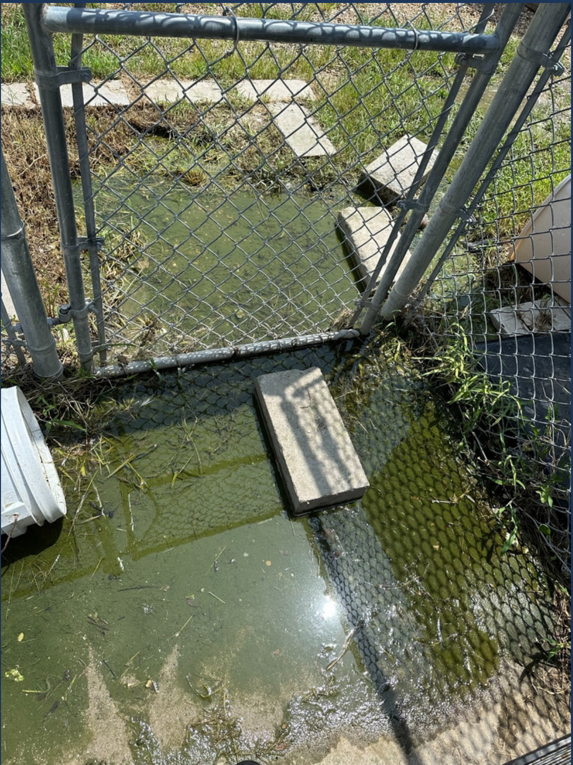
Walkway to Dumpster
