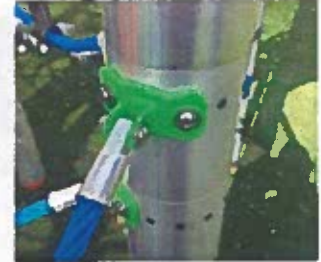
Direct bolt = shear loading at only two attachment points
