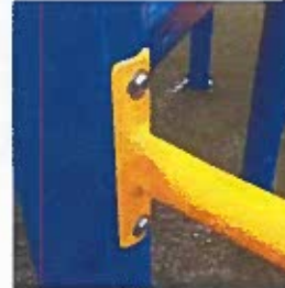
Direct bolt = shear loading at only two attachment points
