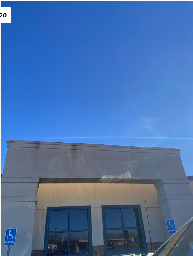
Project: 29961 2031 South Spring Valley Road Date: 12/4/2024, 9:50am Creator: Jacob Yates
