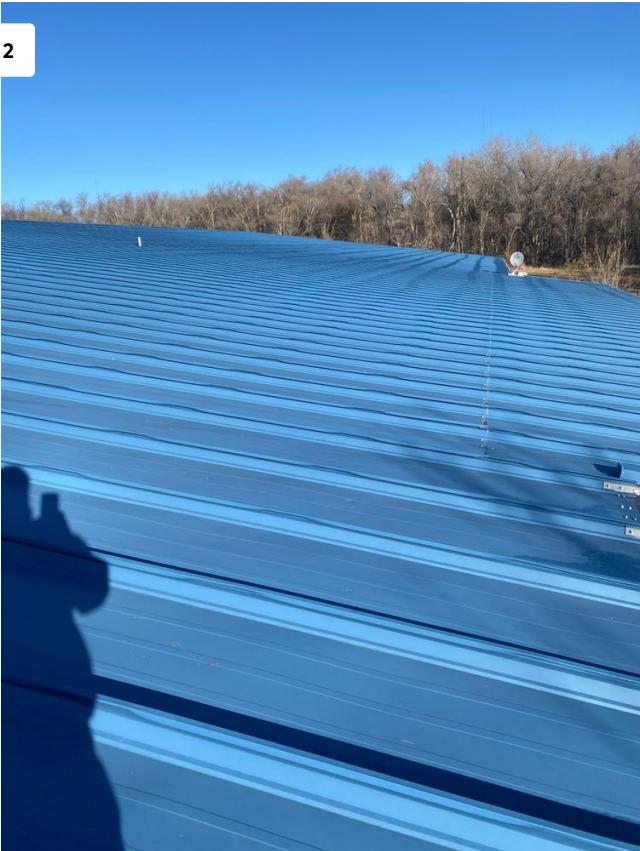
Project: 29961 2031 South Spring Valley Road Date: 12/4/2024, 9:35am Creator: Jacob Yates
