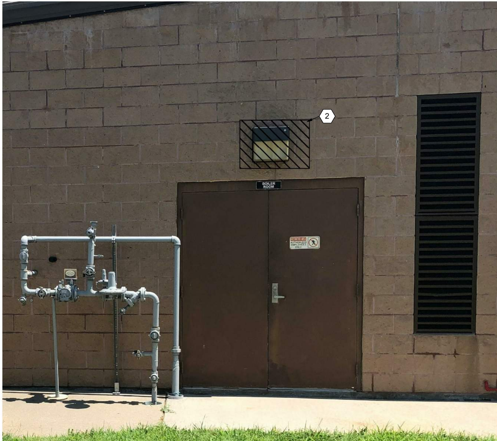
5 BOILER ROOM DEMOLITION PHOTO 213X102 NOT TO SCALE
