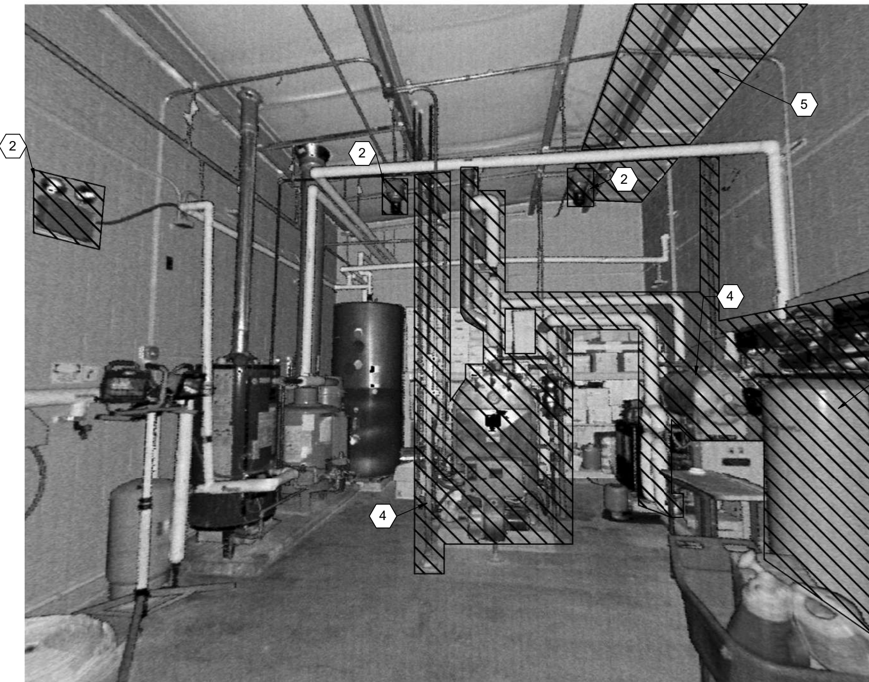
4 BOILER ROOM DEMOLITION PHOTO 213X102 NOT TO SCALE
