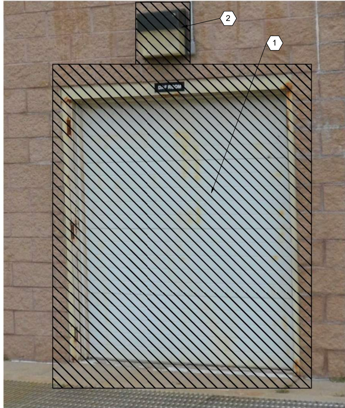
6 DAF ROOM DEMOLITION PHOTO 213X102 NOT TO SCALE
