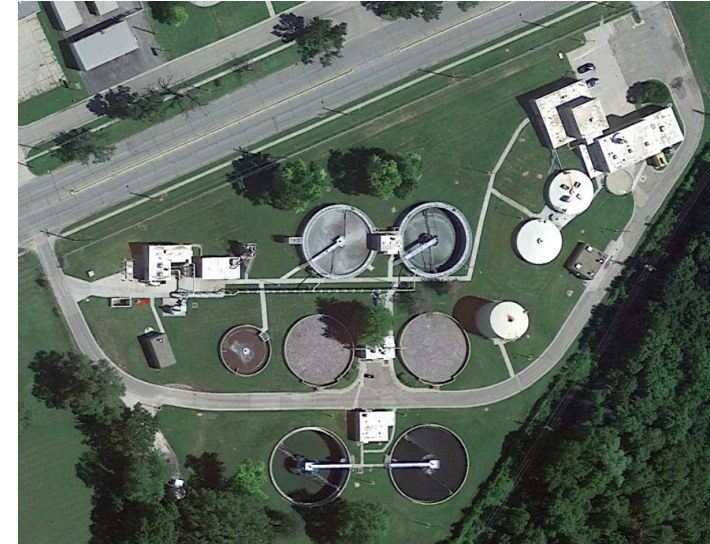
East Wastewater Treatment Plant
