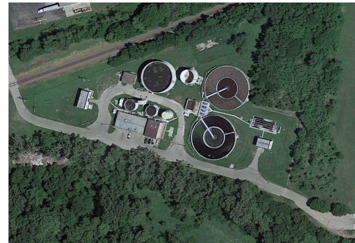
Southwest Wastewater Treatment Plant
