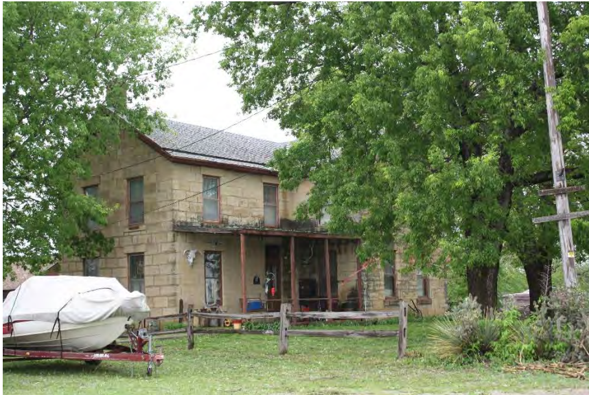
2026 Jackson Street looking northwest from drive showing east and south elevations of stone residence.
