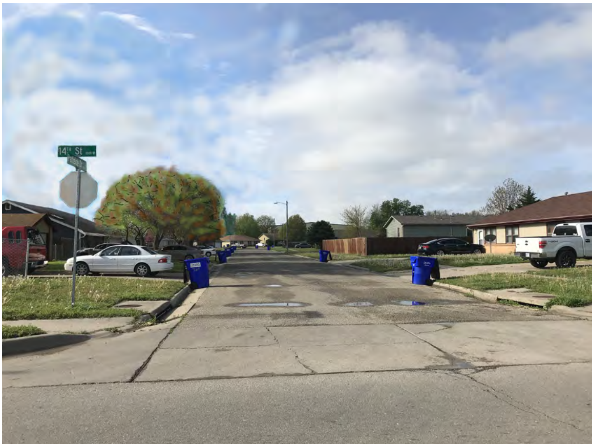
Representative view of neighborhood with large tree removed.
