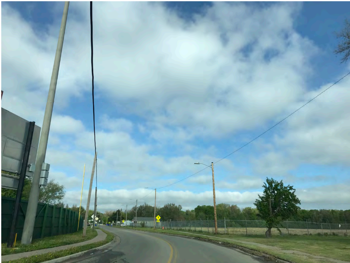
View of utility poles near Runway 36 end.
