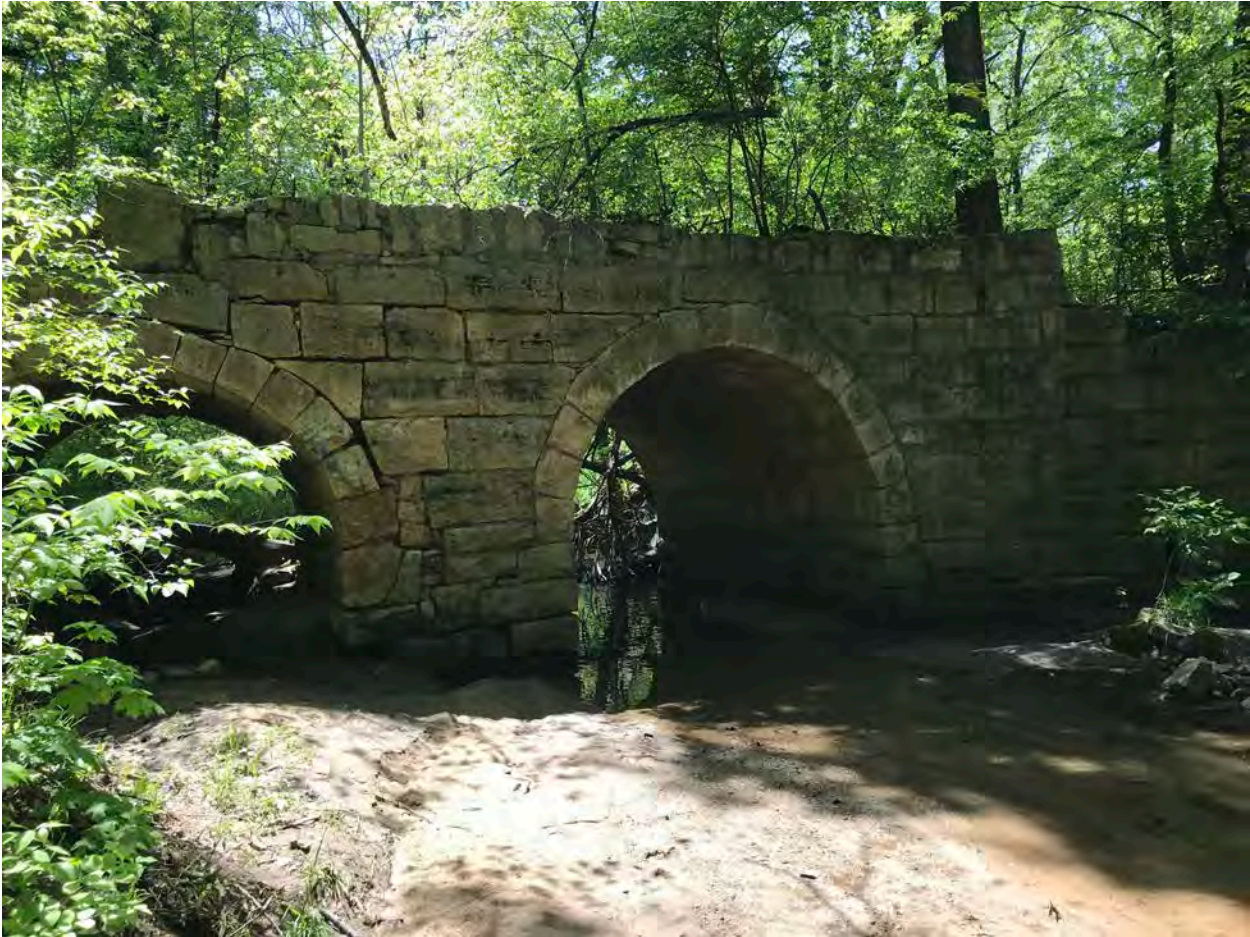
View looking south to bridge – Stream flowing to north from bridge
