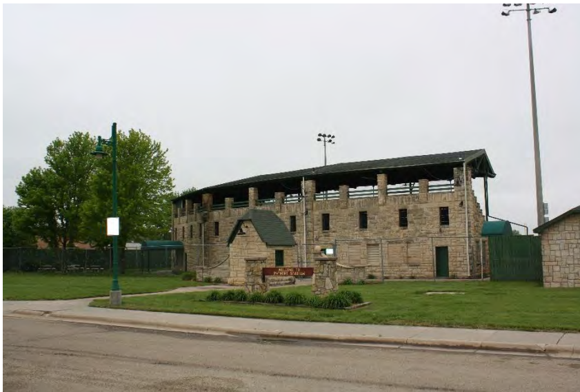
Rathert Stadium and entry gate looking northwest. June 2019.
