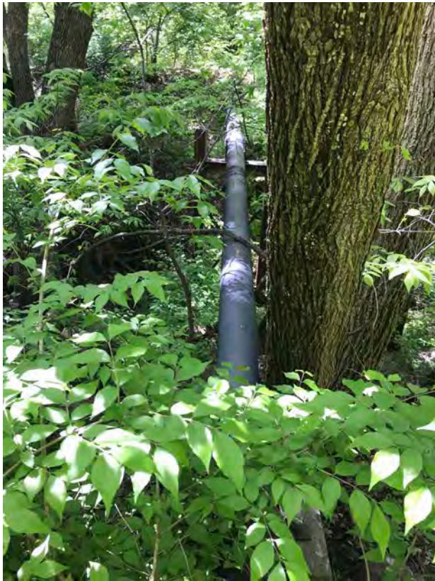
Sanitary sewer force main crossing grade of bridge
